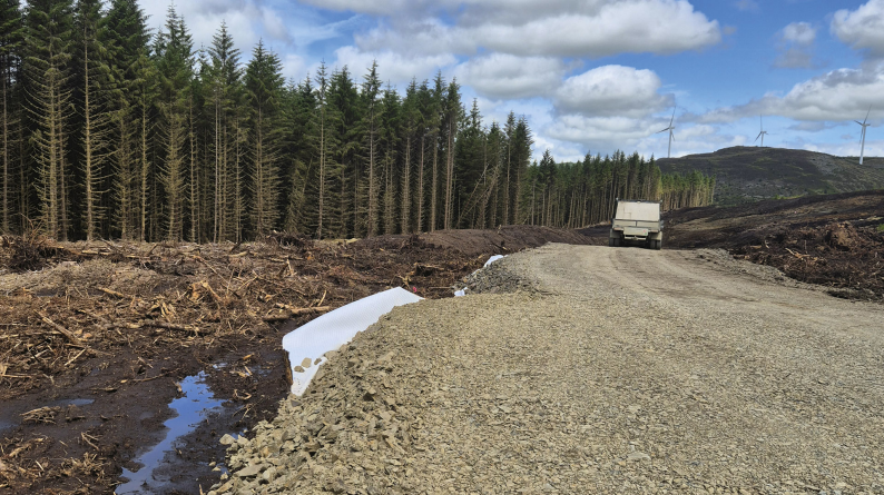
Fig. 1: Naue Combigrid® creates a strong, rigid floating access road
