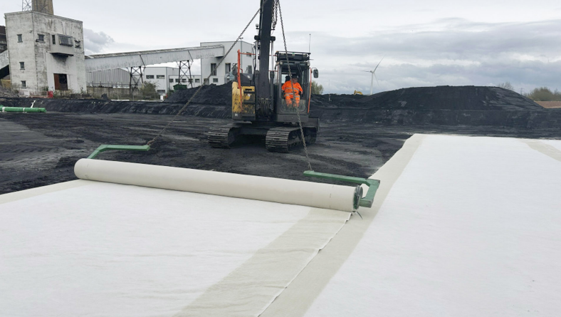
Fig. 1: Installation of Bentofix®
