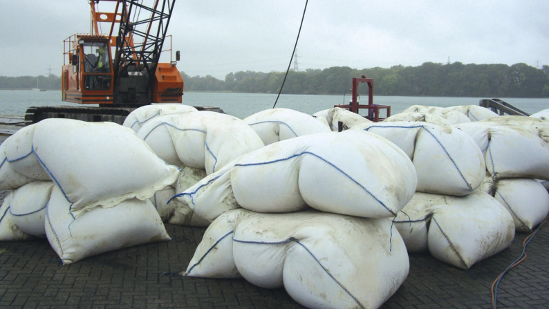
Fig. 1: Storage of sand containers at the terminal
