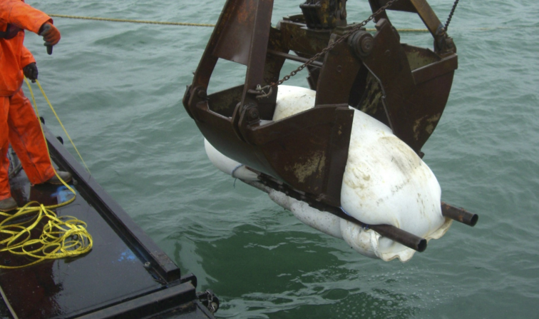
Fig. 2: Installation of Secutex® Soft Rock sand containers
