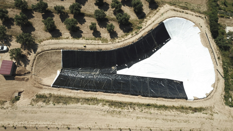
Fig. 1: Installation Naue Carbofol® on top of Secutex® nonwoven
