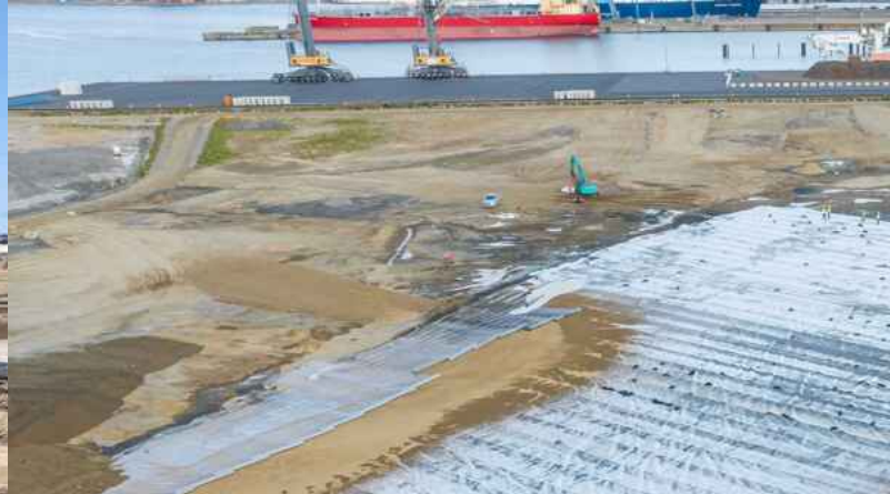
Pic. 2: Aerial view of Secugrid® installation
