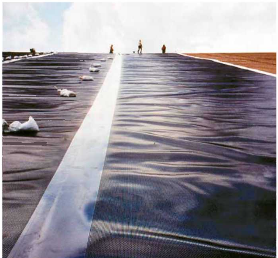
Figure 7 | Structured drain profile on a slope prior to geotextile/cover soils placement
