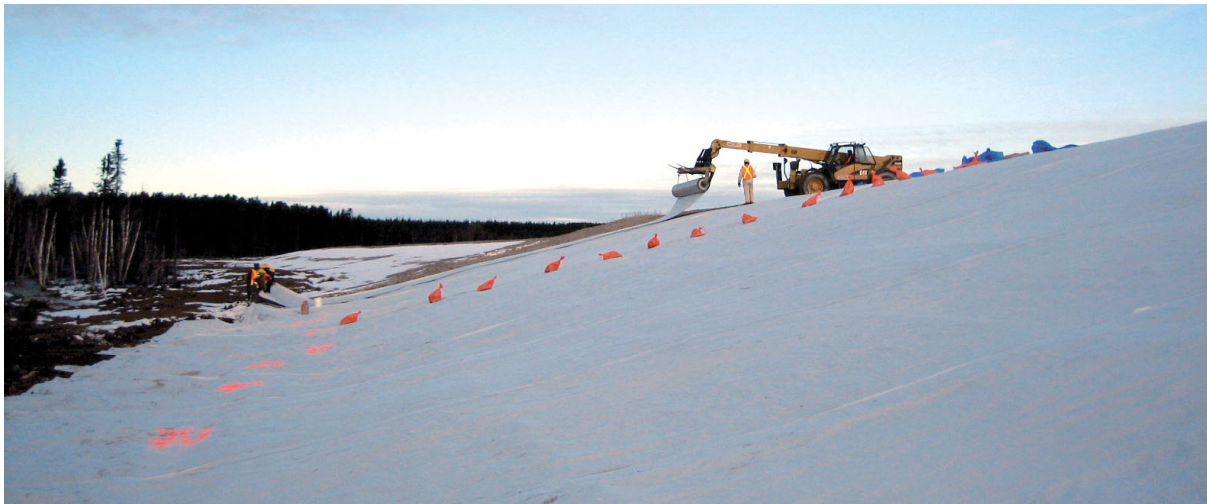
Figure 6: Landfill cap sealed with needlepunched and coated GCL
