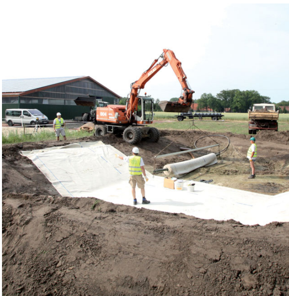
Figure 2: Pond being sealed with a needlepunched and coated GCL
