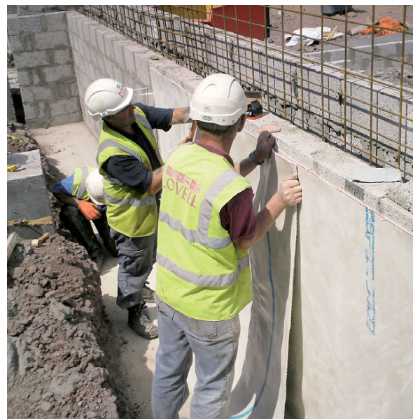
Figure 3: Underground waterproofing sealed with a needlepunched and coated GCL
