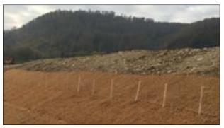
Figure 4: Coir net to be fixed with a wooden pin
