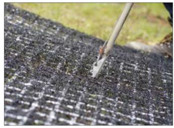
Figure 5: Loadlocking and tensioning the earth anchor
