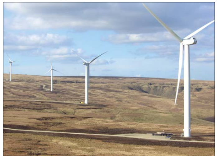
Fig. 4 Finalised windfarm with Secugrid® soil reinforced areas
