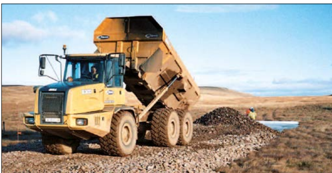
Fig. 3 Placement of aggregate on Naue Secugrid®
