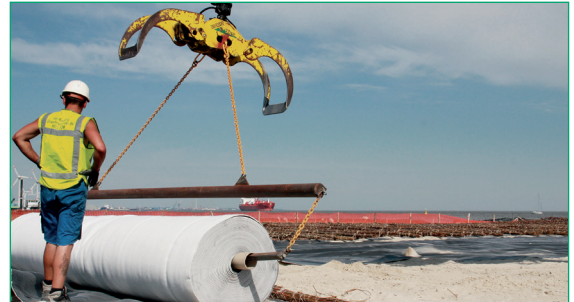
Figure 8 Secutex® H installation
