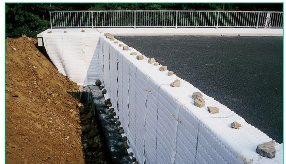
Figure 9 Secudrain® installation
