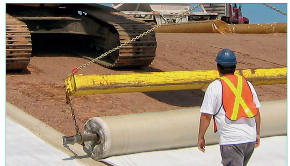
Figure 6 Bentofix® installation
