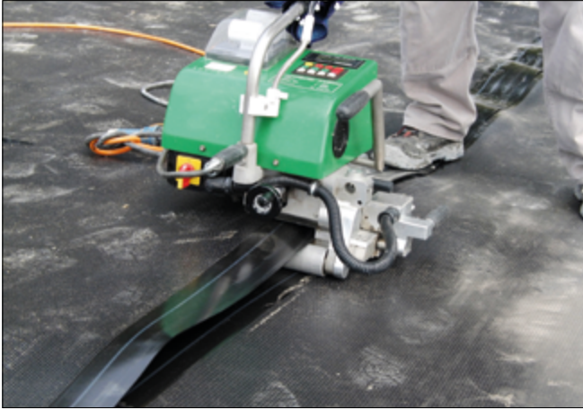
Figure 1: Welding machine in operation on Carbofol®
