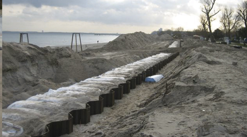
Fig. 2: Geotextile sand container as scour protection for sheet pile wall
