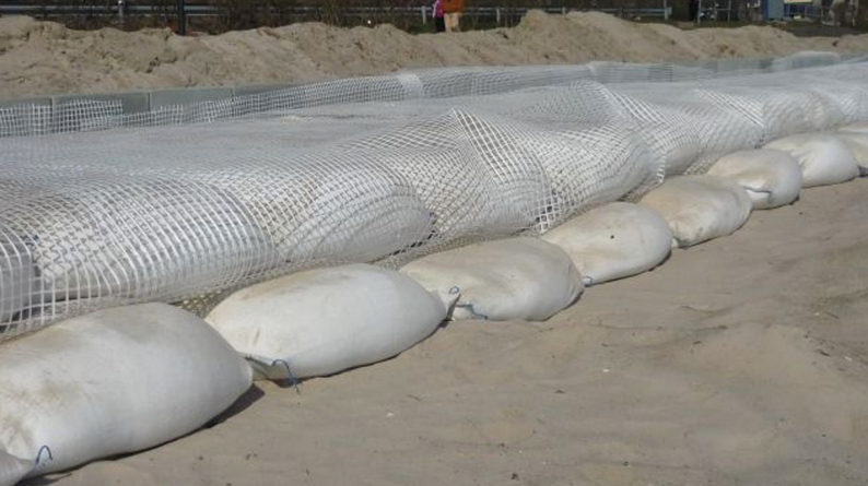
Fig. 1: Top sand container layer wrapped with Secugrid® 30/30 Q1
