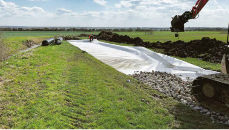
Pic. 1: Installation of base course on top of Combigrid®
