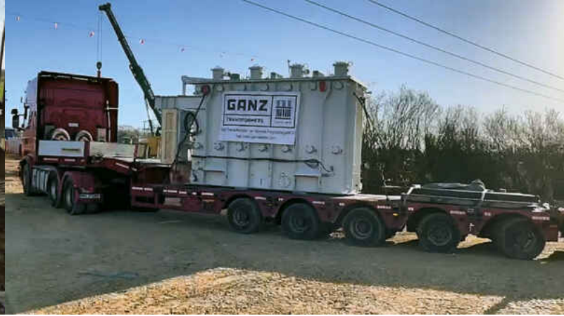
Pic. 2: Flat-bed trailer on access road
