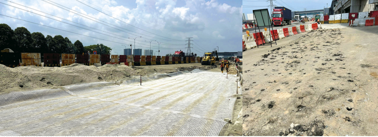
Fig. 1: Secugrid® as base course reinforcement
