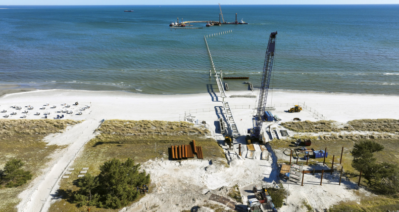
Fig. 1: Construction of the pier
