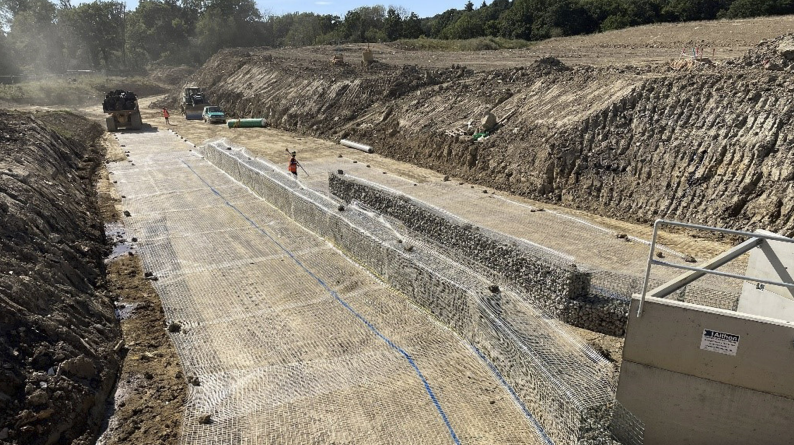
Fig. 1: Installation of Naue Secugrid®
