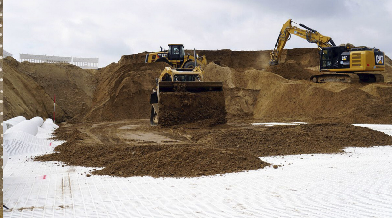
Fig. 2: Installation of the cover layer (above the geogrid)
