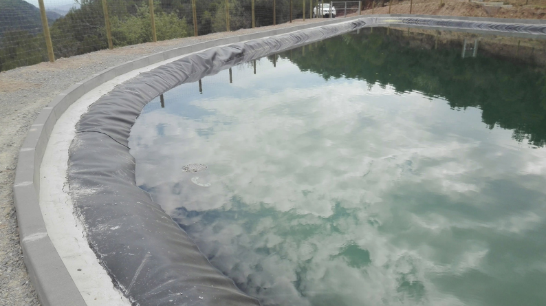
Fig. 2: Retention basin before using Naue Secumat® for passage
