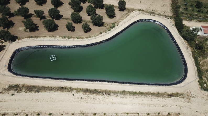
Fig. 2: Top view on irrigation pond
