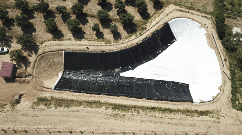
Fig. 1: Installation Naue Carbofol® on top of Secutex® nonwoven
