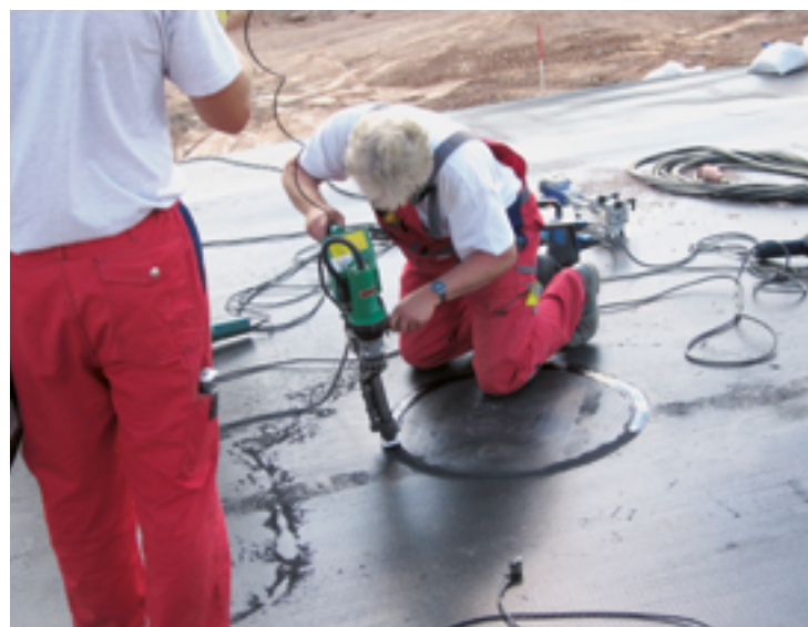
Figure 1: Welding on-site is improved by the high melt flow rate
