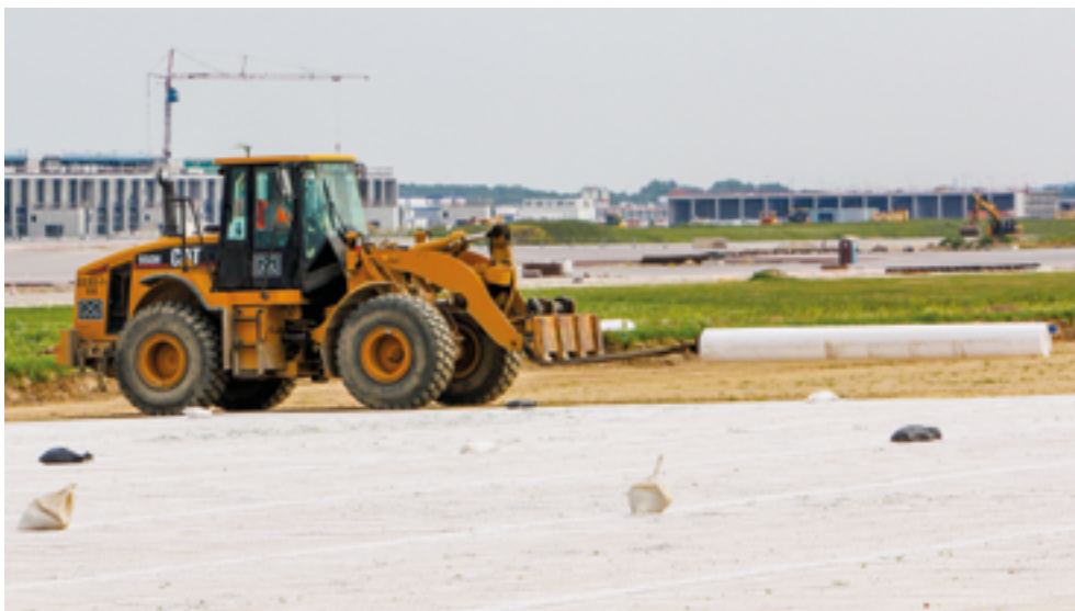
Figure 11: Installation of Secugrid® (no pre-stressing required)
