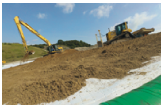
Figure 18: Secudrain® BAM used in a landfill capping system between the surface liner and the cover soil layer
