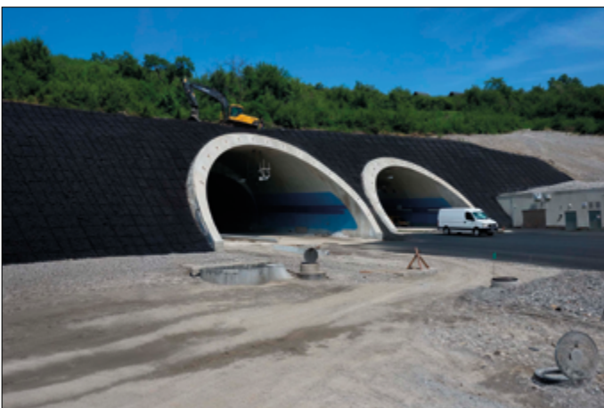
Secumat® erosion control mat on a tunnel embankment
