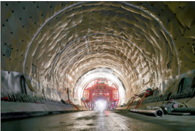
Bentofix® X type in the arch area
