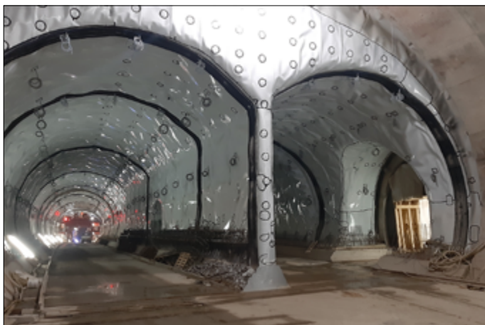
Carbofol® tunnel sealing with Carbofol® ME Anchor
