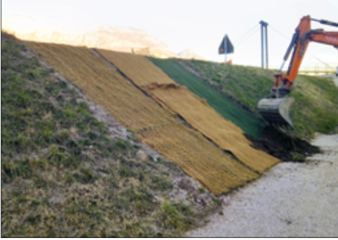
Figure 6: Secumat® Green 3D Mesh on a riverbank (inland side)
