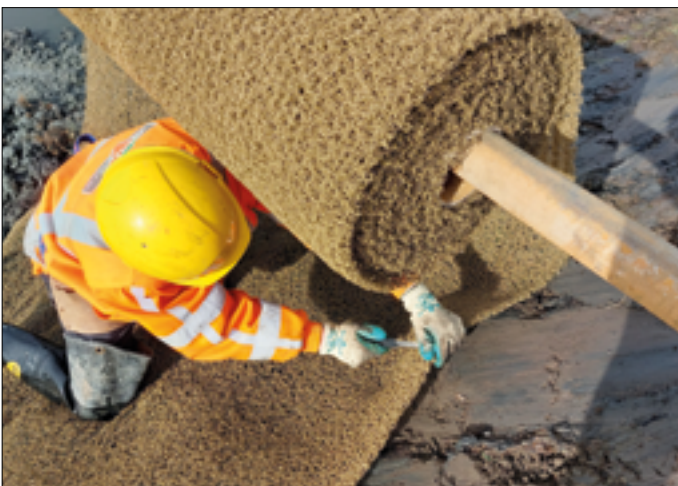
Figure 8: Secumat® Green 3D Mesh on a stream bank
