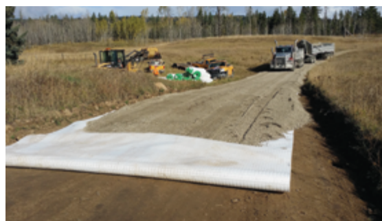
Figure 7: Combigrd® and Secugrid® installation
