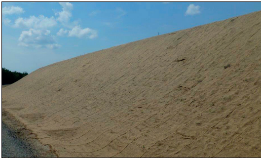
Fig. 1: Slope with Secumat® Green Jute nets
