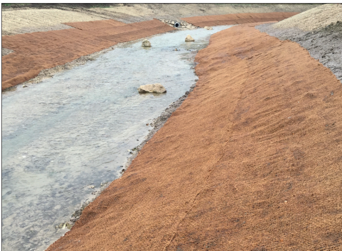
Figure 8: Coir nets in trenches and brooks
