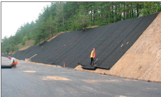
Fig. 3: Road slope with Secumat® geomats
