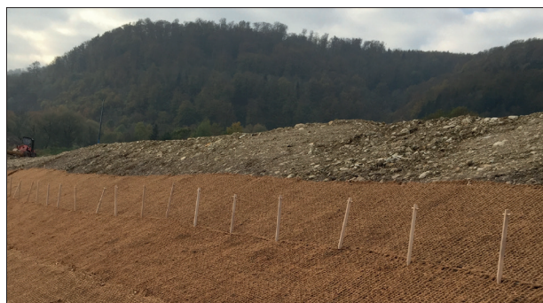
Figure 4: Coir net to be fixed with a wooden pin
