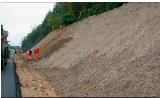
Fig. 2: Levelling of road embankment surface
