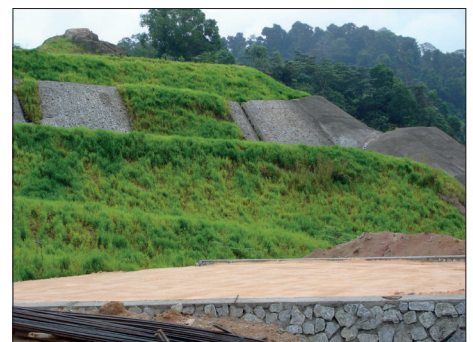
Figure 6: Erosion control vegetated
