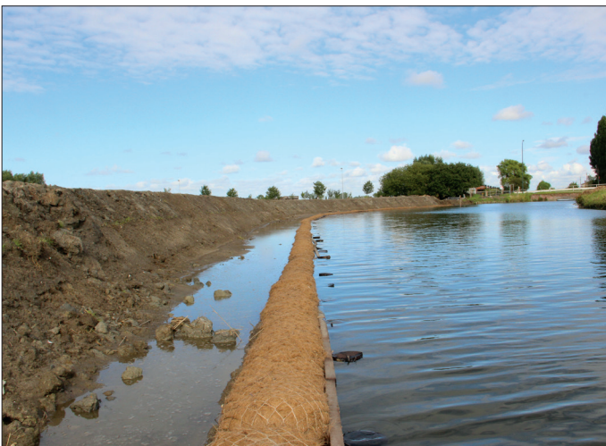
Figure 8: Georolls in a trench
