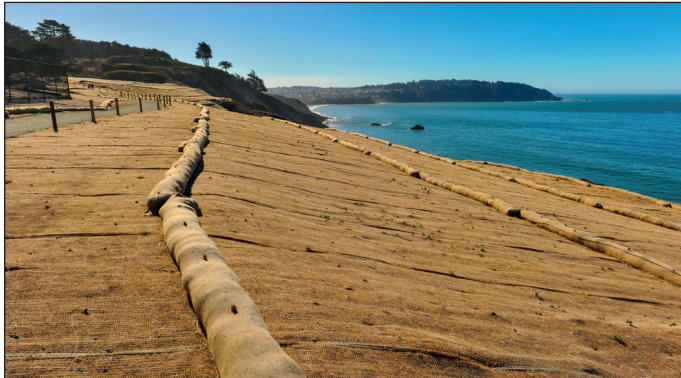
Fig. 5 Georolls on a slope
