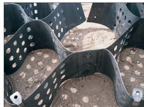
Figure 6: Secumat® Cell 150 geocell high screwed together with Secumat® Screw and fixed to the soil with Secumat® PinCap
