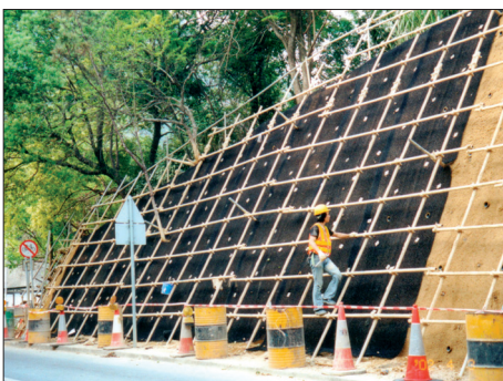
2 Figure 1: Erosion control on street slopes
