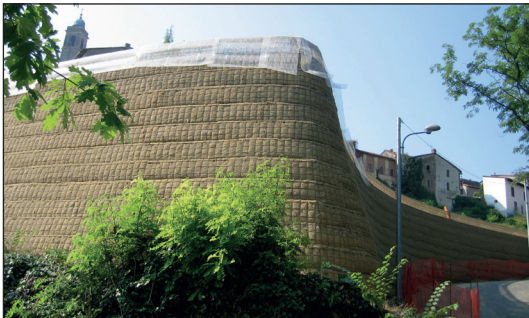
Fig. 2: Soil reinforced with Secumat® Green coirmats
