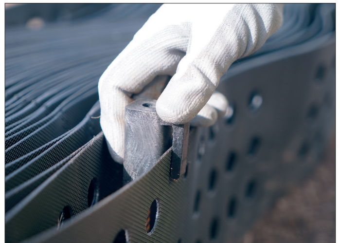
Figure 10: Inserting Secumat® PinCap
