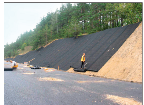
Figure 3: Secured highway slopes
