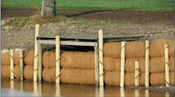
Fig. 4 Stacked georolls on the cut embankment of a trench
