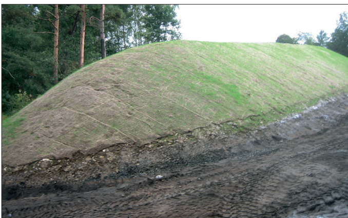
Figure 8: Jute nets on a slope
