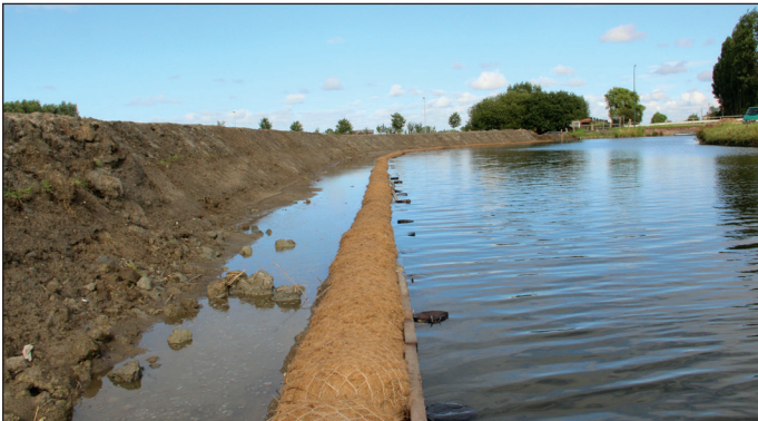
Fig. 3 Georolls on the bank of a body of water
