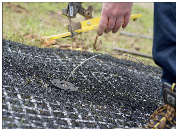
Figure 5: Loadlocking and tensioning the earth anchor
