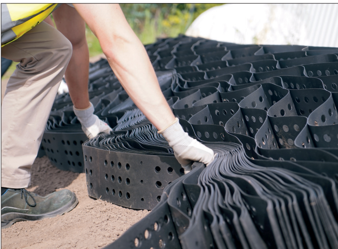
Figure 9: Laying out Secumat® Cell 150 on a slope
