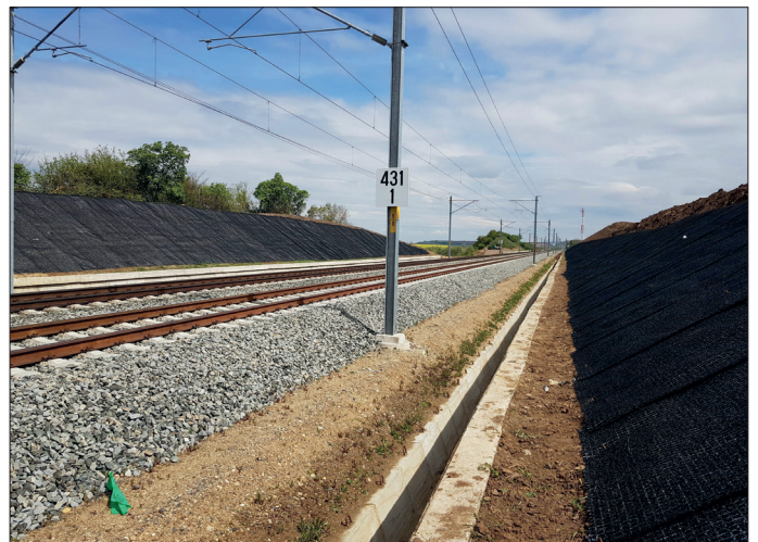
Figure 22: Rail slope with 3D Mesh
