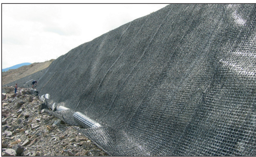
Fig. 2: Installation of Naue Clamp system
