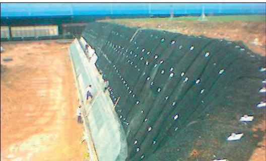
Fig. 2: Installation of Naue Nail system
