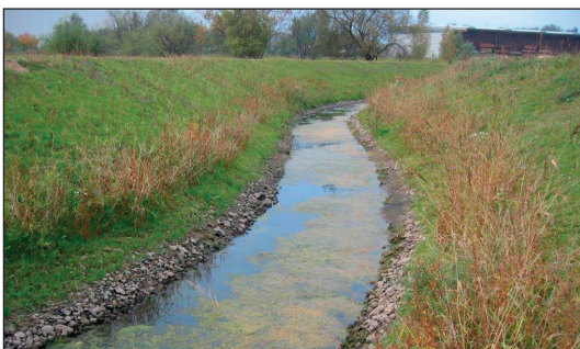
Fig. 4: Trench bank with Secumat® combined geomats
