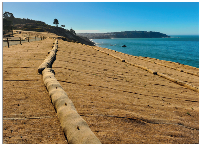
Figure 9: Georolls parallel to the slope
