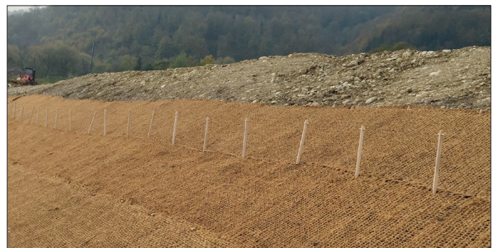
Figure 5: Installing the coir net with wooden fixings
