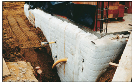
Figure 65 Backfilling against Secudrain® system
