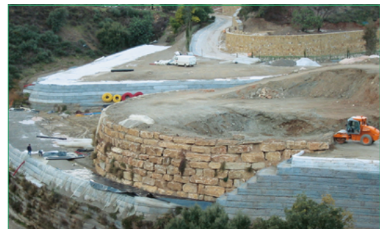
Figure 55 Construction of a retaining wall using Secugrid® (Marbella Hill, Spain)
