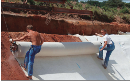
Figure 33 Installation of Bentofix® with a spreader bar in a road ditch (Muenster, Germany)
