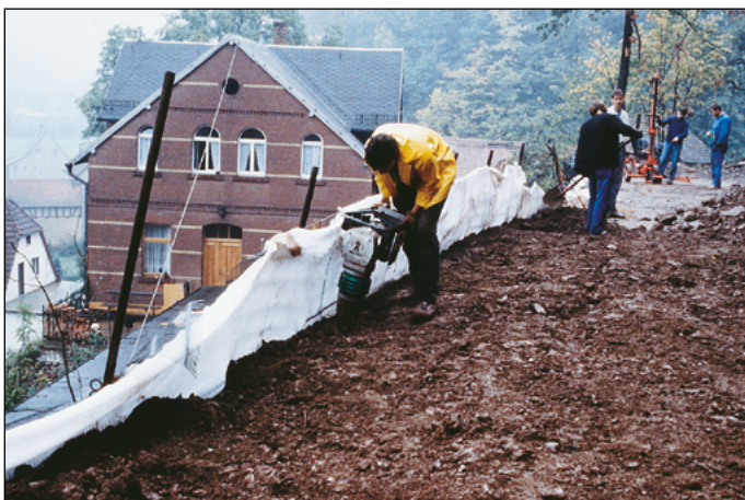
Figure 6 Secutex® as a geotextile filter in a retaining wall to prevent the washing out of fines at the front face
