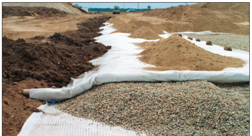
Figure 9 Secutex® separates the gravel drainage layer from the silty subsoil
