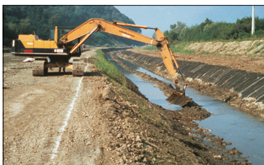
Figure 50 Soil coverage of Secumat® for erosion control in a rainwater collector (Albertville, France)
