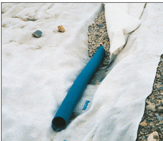
Figure 8 The side rainwater collection pipe and drain is wrapped with a Secutex® geotextile to prevent fines from clogging the drain
