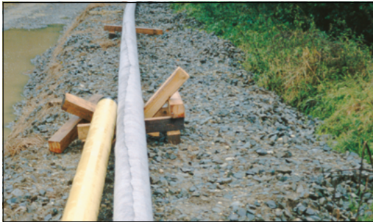
Figure 82 Protection wrapping of a pipeline with Secutex® (Armstorf, Germany)
