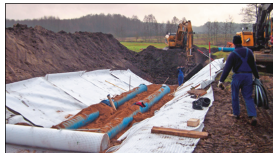
Figure 83 Increasing the soil bearing capacity in a pipe ditch with Combigrig® (Briesen, Germany)
