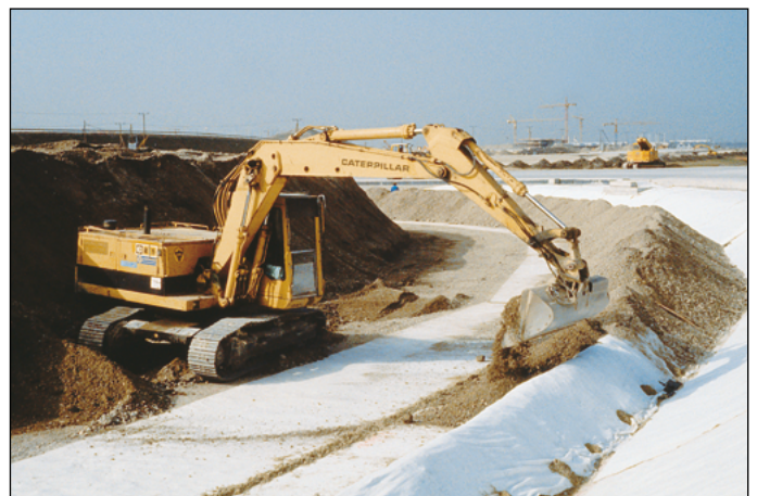
Figure 7 Secutex® geotextile filter ensures that the fines are not washed out of the filter dam
