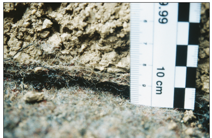
Figure 12 In-situ measured thickness of Secudrain® after over 12 years with a confining stress of 1.20m cover soil
