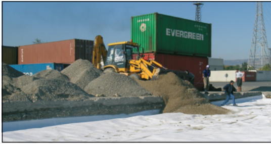
Figure 19 Combigrid® increasing the soil bearing capacity (Mersin, Turkey)
