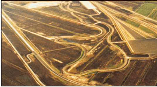
Figure 15 Separation and filtration with Secutex® in a car testing track (Papenburg, Germany)
