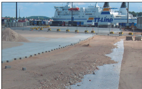
Figure 29 Pre-stressed Secugrid® installed under a base course for heavy traffic (Luebeck, Germany)
