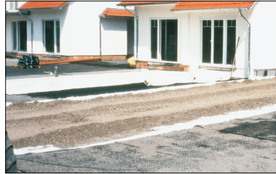
Figure 26 Separation and filtration with Secutex® in a driveway (Gehlenbeck, Germany)
