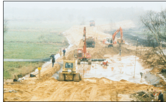
Figure 16 Use of Secugrid® for a dam reinforcement (Loxstedt, Germany)
