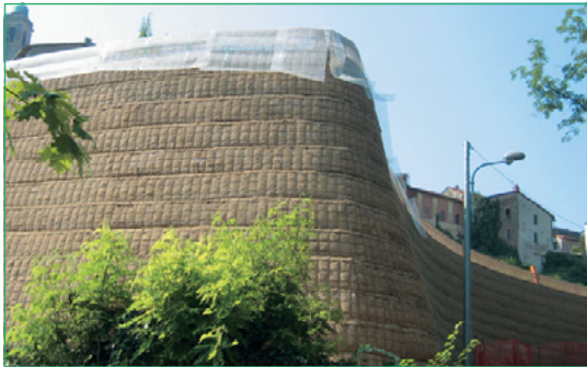
Figure 54 Secugrid® reinforced earth wall (Vignale, Italy)
