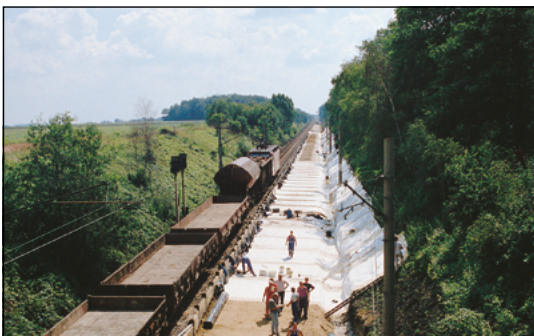
... in the construction of transportation routes to seal the subgrade in sensitive groundwater protection areas ...
