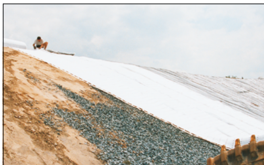
Figure 49 Slope stabilisation and collection of see- page water with Secudrain®
