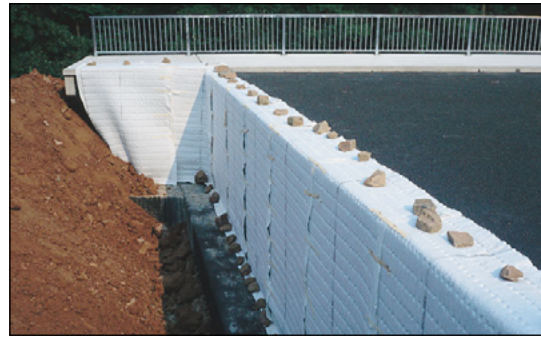
Figure 70 Installed Secudrain® on a bridge structure (Grossen-Marpe, Germany)
