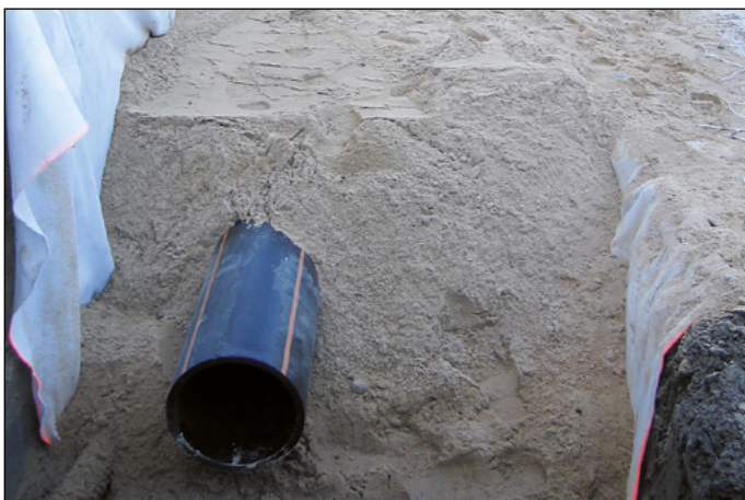
Figure 1 Secutex® used as separation geotextile between a pipe bedding and the silty subsoil
