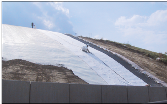
... on steep slopes to improve slope stability and erosion control, ...
