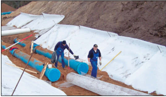
Figure 86 Installation of Combigrd® to increase the pipe foundation (Wismar, Germany)
