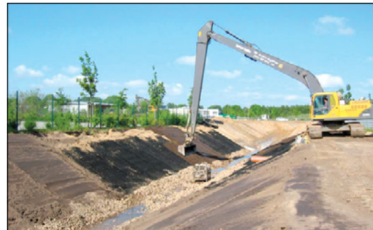
Figure 46 Erosion control on a slope. The open pore structure of Secumat® allows easy filling of the top soil
