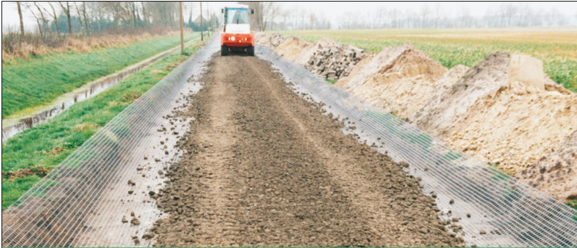
Naue geosynthetics may be used in various system solutions, such as in road construction to increase the bearing capacity and to reduce rutting ...
