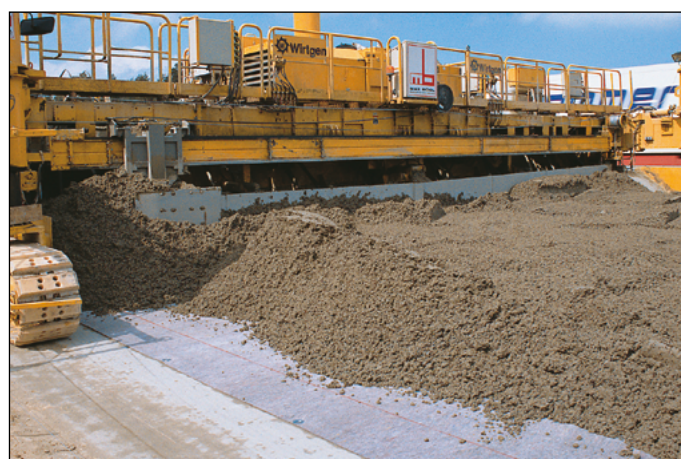
Figure 4 Concrete placement over Secutex®, which acts as a separator, filter and drainage layer between the subsoil and the road
