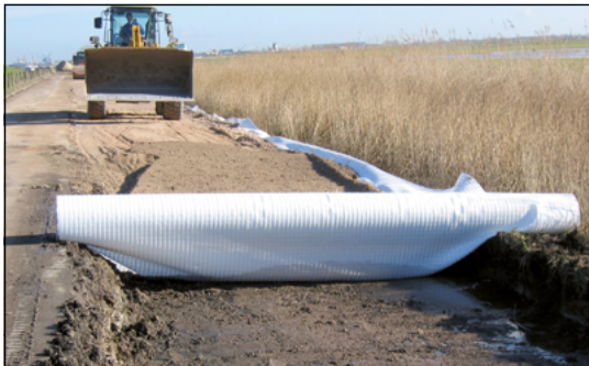
Figure 25 Installation of Combigrig® to increase the soil bearing capacity (Bremerhaven, Germany)
