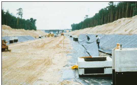
Figure 39 Carbofol® geo- membranes in a groundwater sensitive area (UK)
