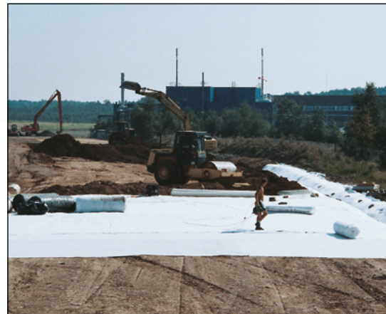
Figure 34 Installation of Bentofix® GCL as groundwater protection under the B 82n highway (Langelsheim, Germany)
