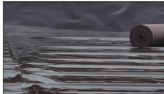
Figure 75 Welded Carbofol® geomembrane (Allmannsweiler, Germany)
