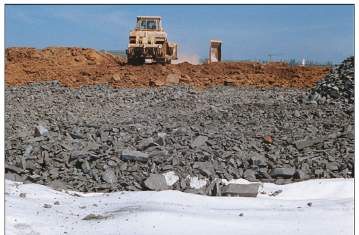
Figure 2 The high elongation capacity of Secutex® ensures excellent damage resistance
