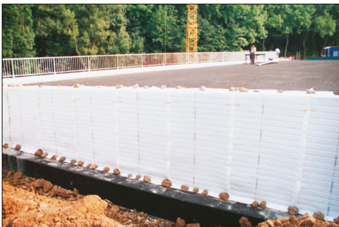
Figure 11 Secudrain® in a bridge abutment ensuring long-term drainage
