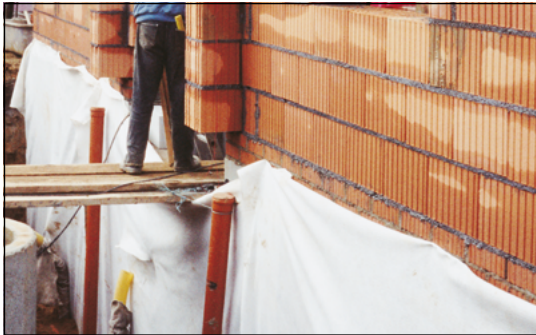
Figure 63 Secudrain® basement drainage and protection layer to waterproofing membrane
