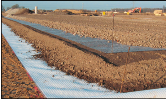
Figure 73 Placing of cover soil over the Combigrig® and Secugrid® reinforced structure (Nordenham, Germany)
