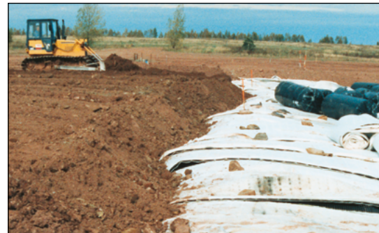
Figure 79 Two layers of Secugrid® reinforcement as base course reinforcement of a federal road (Loxstedt, Germany)
