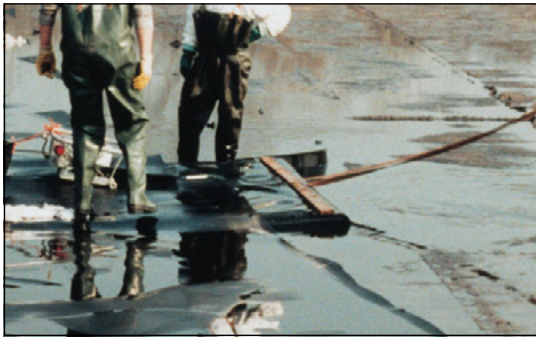
Figure 78 Welding of the gas barrier Carbofol® on a sludge pond (Rositz, Germany)
