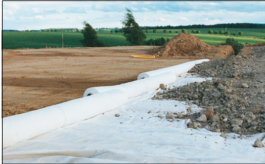
Figure 24 Secutex® as a separation geotextile between fine and coarse grained soils
