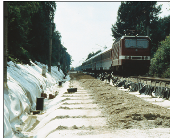
Figure 40 Use of Bentofix® GCL under railway tracks for groundwater pro- tection (Dresden to Leipzig, Germany)
