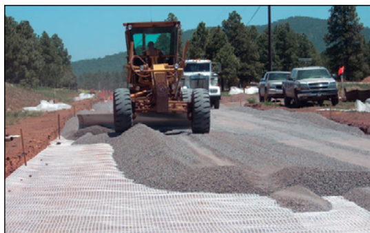
Figure 30 Soil coverage of Secugrid® reinforcement in a base course (Arizona, USA)
