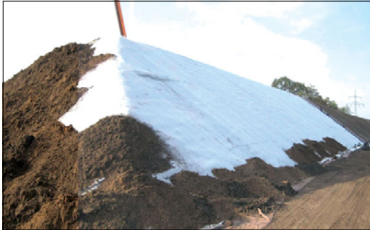
Figure 44 Secugrid® ensures the slope stability on a noise barrier dam (A33 Bielefeld, Germany)
