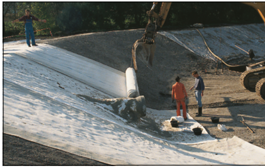
Figure 38 Bentofix® GCL installation in a stormwater retention pond
