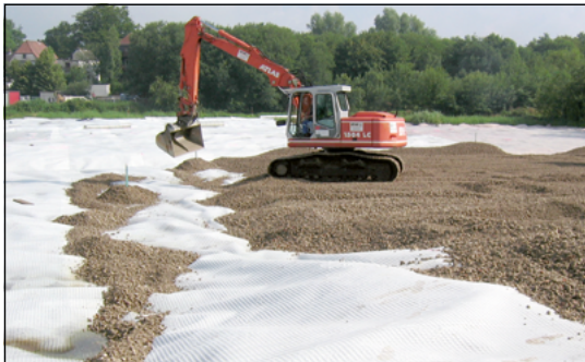
Figure 74 Soil placement over Combigrig® and an extreme weak soft soil (Germany)
