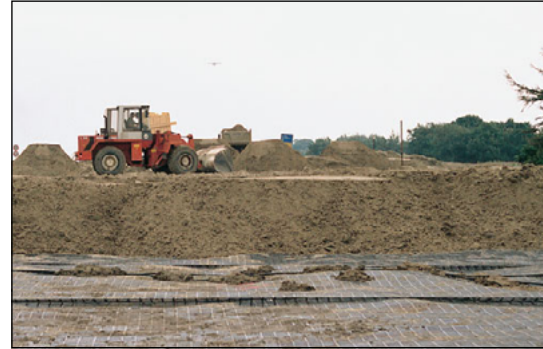
Figure 21 Prevention of soil failure with Secugrid® 400/60 R 6 (A 31, Emden, Germany)
