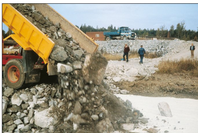
Figure 3 Secutex® nonwoven geotextiles can resist high dynamic installation forces
