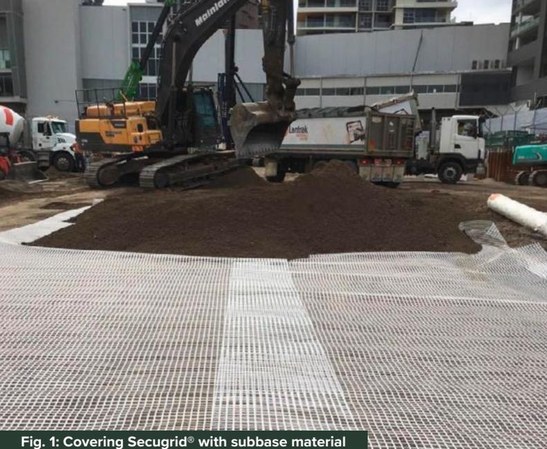
**Fig. 1: Covering Secugrid® with subbase material**
