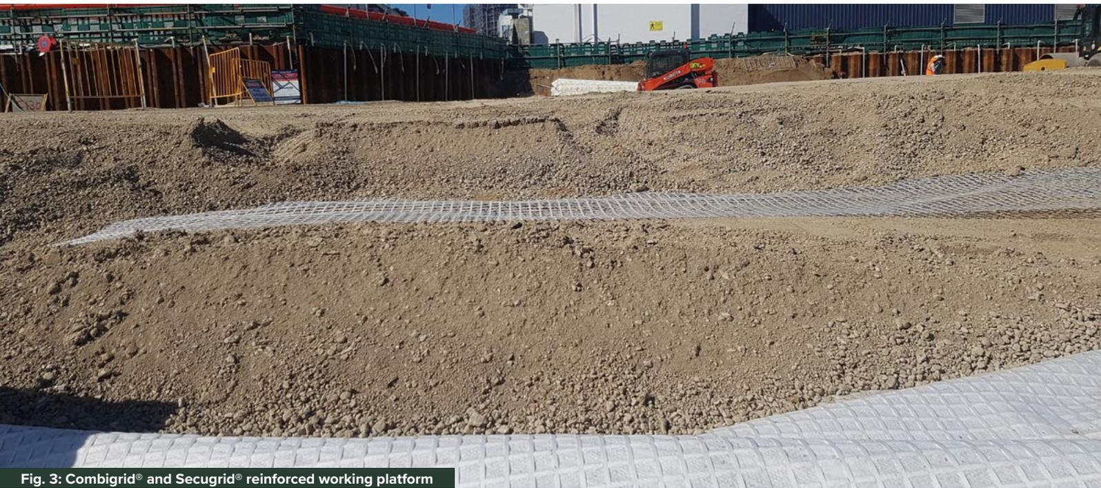
**Fig. 3: Combigrid® and Secugrid® reinforced working platform**
