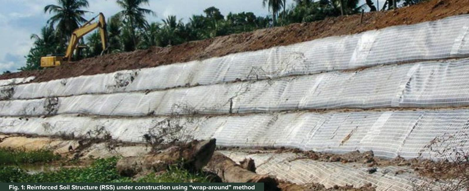
**Fig. 1: Reinforced Soil Structure (RSS) under construction using “wrap-around” method**
