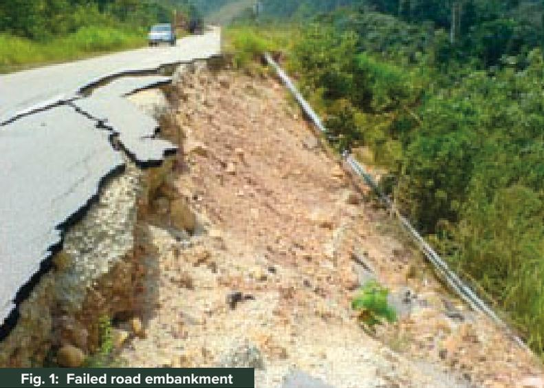
Fig. 1: Failed road embankment
