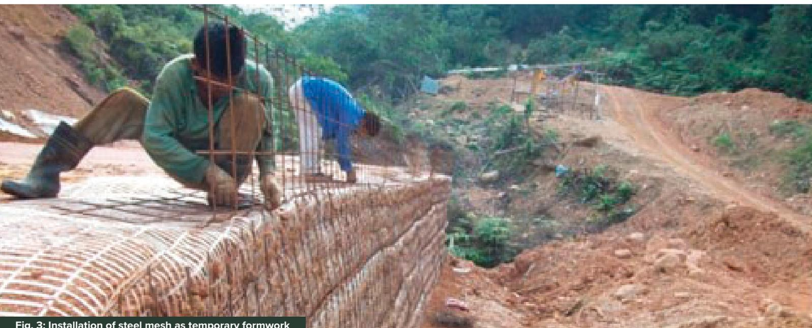
Fig. 3: Installation of steel mesh as temporary formwork
