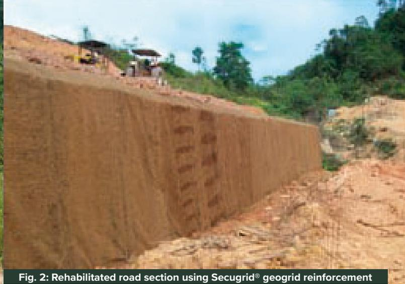
Fig. 2: Rehabilitated road section using Secugrid® geogrid reinforcement
