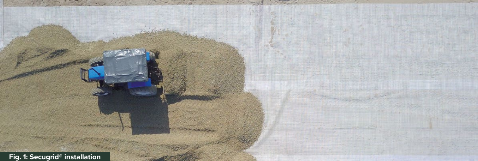
Fig. 1: Secugrid® installation
