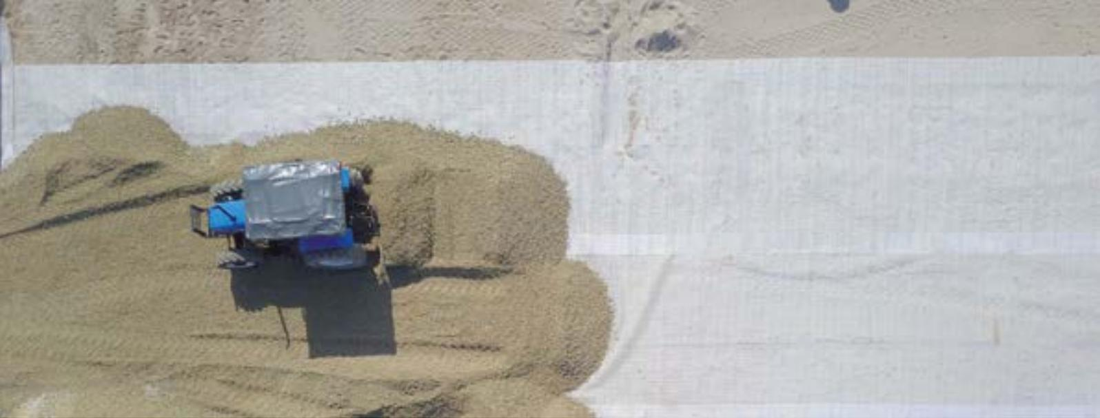
Fig. 1: Secugrid® installation
