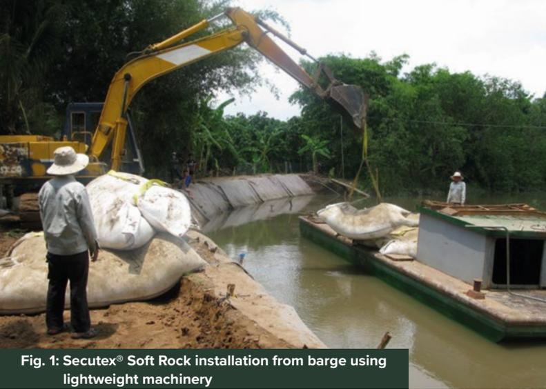
**Fig. 1: Secutex® Soft Rock installation from barge using lightweight machinery**
