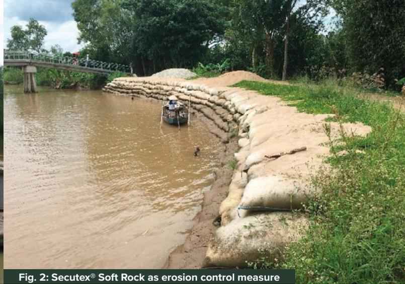
**Fig. 2: Secutex® Soft Rock as erosion control measure**
