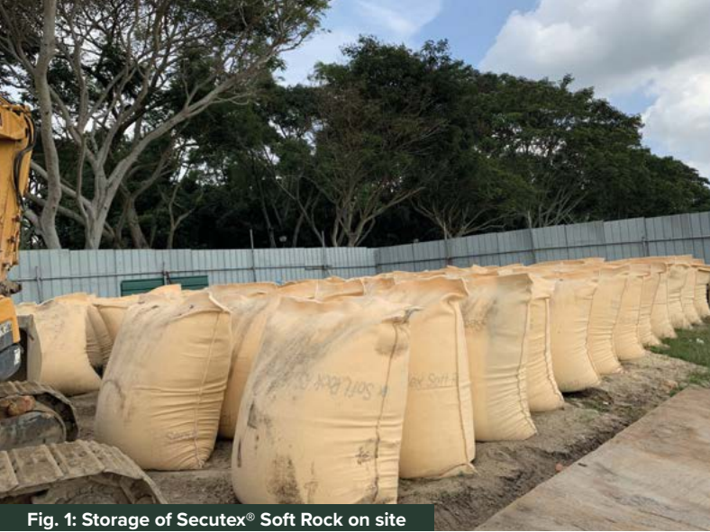
Fig. 1: Storage of Secutex® Soft Rock on site
