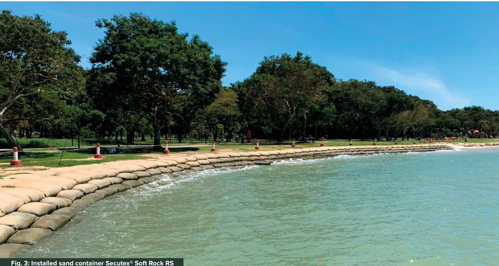
Fig. 3: Installed sand container Secutex® Soft Rock RS
