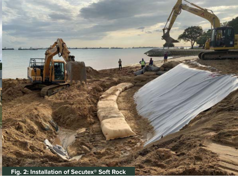
Fig. 2: Installation of Secutex® Soft Rock
