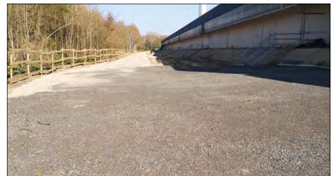
Fig. 2: Completed temporary construction road
