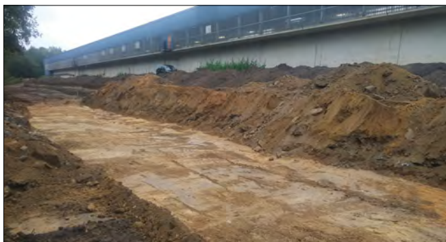
Fig. 1: Prepared subgrade for the construction of a temporary road
