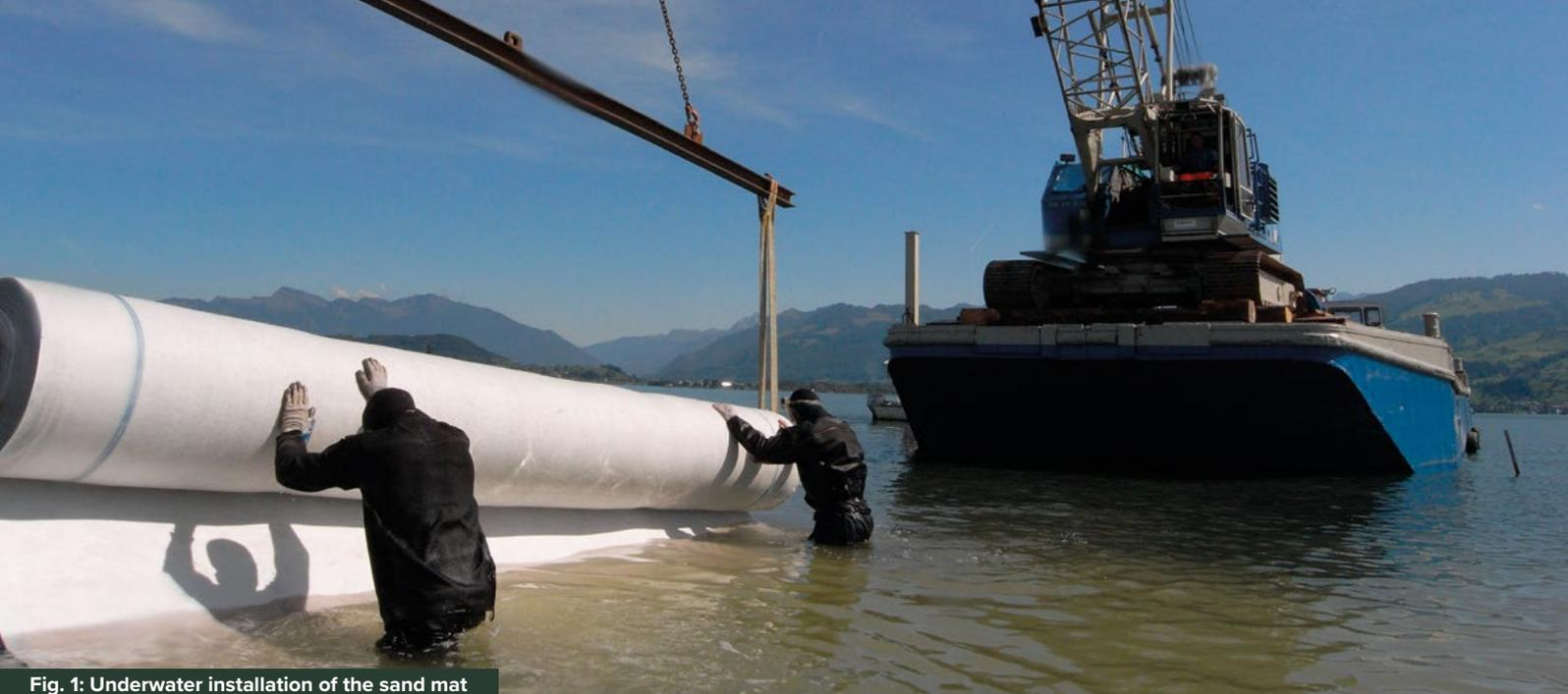
Fig. 1: Underwater installation of the sand mat
