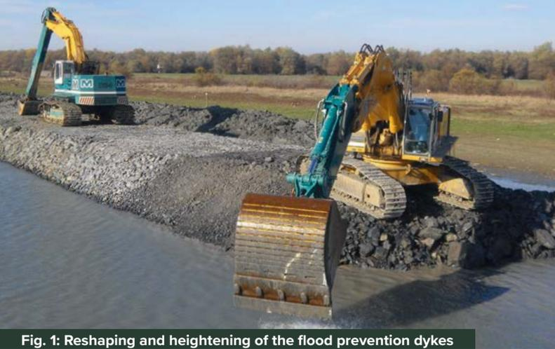
Fig. 1: Reshaping and heightening of the flood prevention dykes
