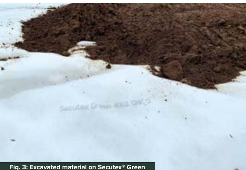
Fig. 3: Excavated material on Secutex® Green
