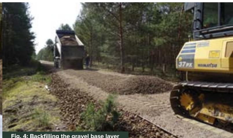
**Fig. 4: Backfilling the gravel base layer**
