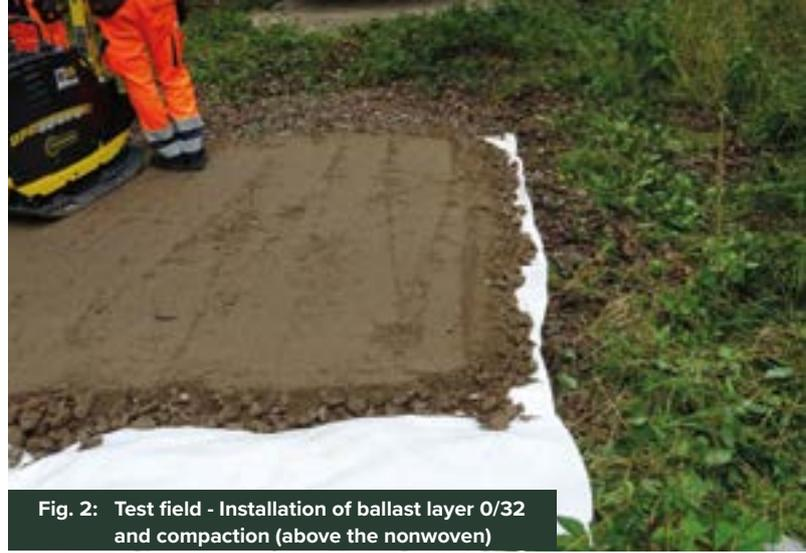
**Fig. 2: Test field - Installation of ballast layer 0/32 and compaction (above the nonwoven)**
