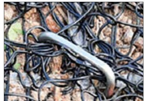
Figure 5: Secumat® 3D Mesh fixed with a steel pin
