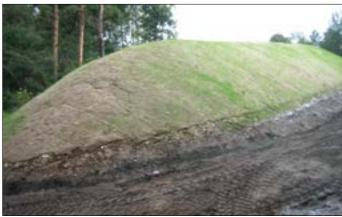
Figure 8: Jute nets on a slope
