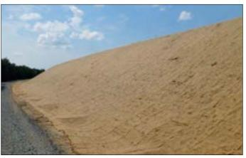
Figure 9: Jute nets as erosion control by a road
