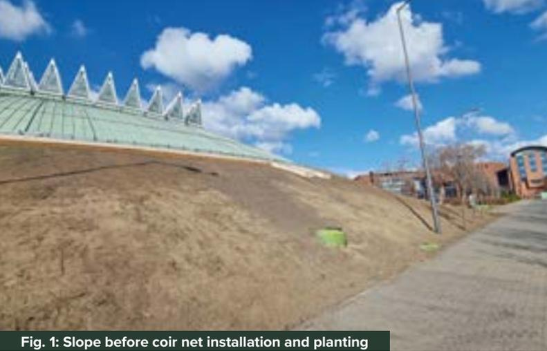
Fig. 1: Slope before coir net installation and planting
