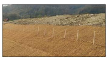
Figure 5: Installing the coir net with wooden fixings
