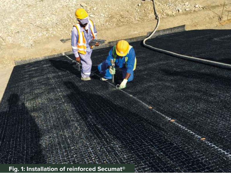
Fig. 1: Installation of reinforced Secumat®
