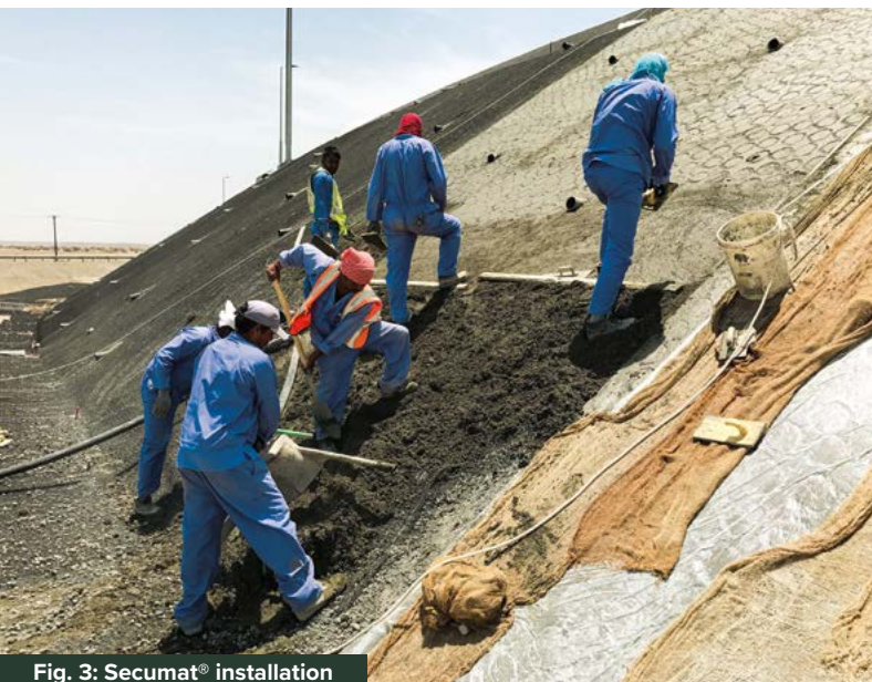
Fig. 3: Secumat® installation
