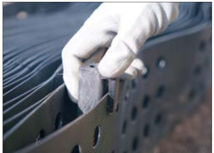
Figure 10: Inserting Secumat® PinCap
