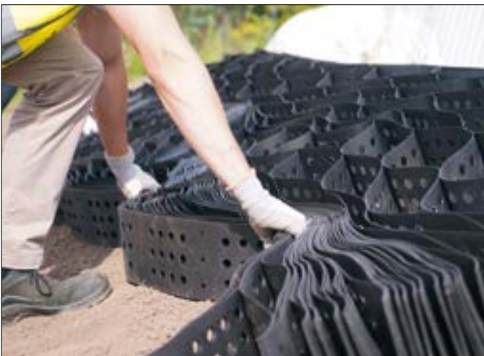
Figure 9: Laying out Secumat® Cell 150 on a slope
