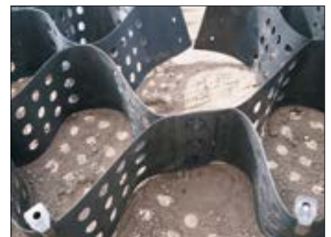
Figure 6: Secumat® Cell 150 geocell high screwed together with Secumat® Screw and fixed to the soil with Secumat® PinCap
