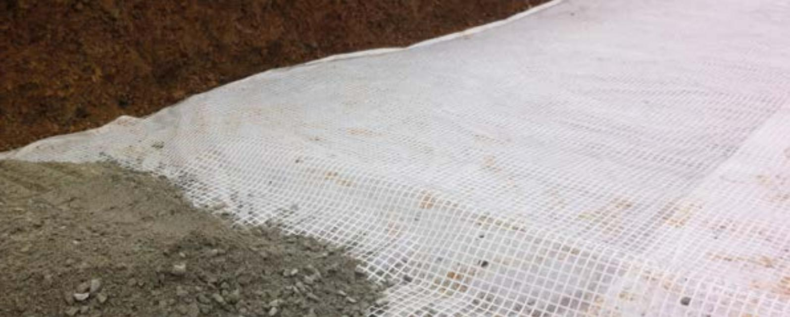
Secugrid® geogrids from Naue proved to be the most cost-effective and technically beneficial solution for the mechanical reinforcement of unbound access roads and crane pads.
