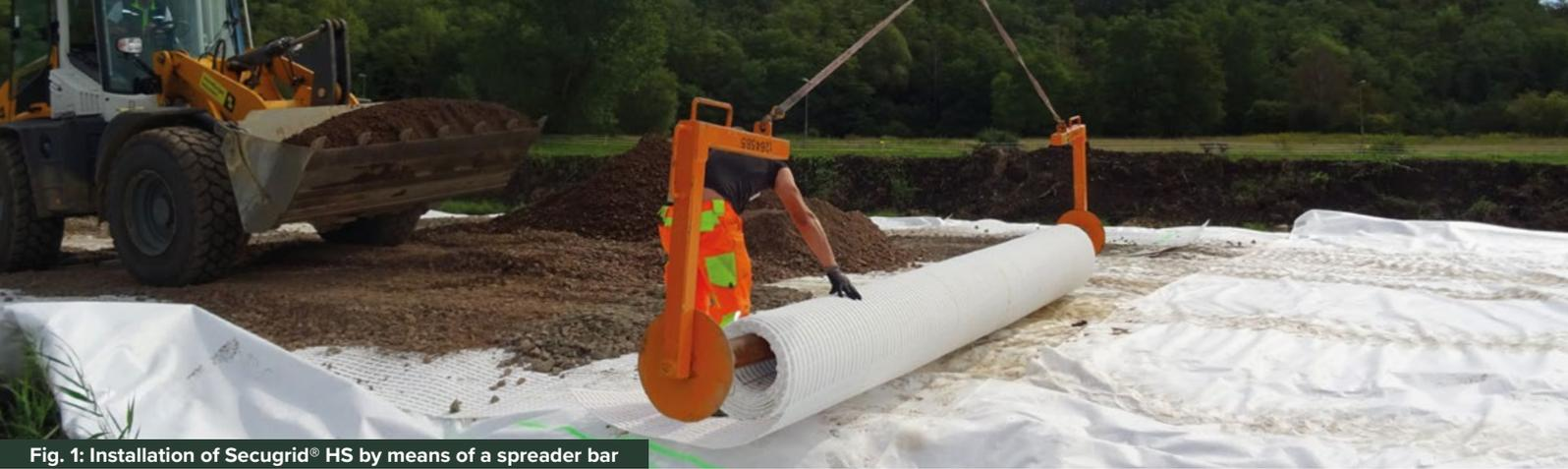
**Fig. 1: Installation of Secugrid® HS by means of a spreader bar**
