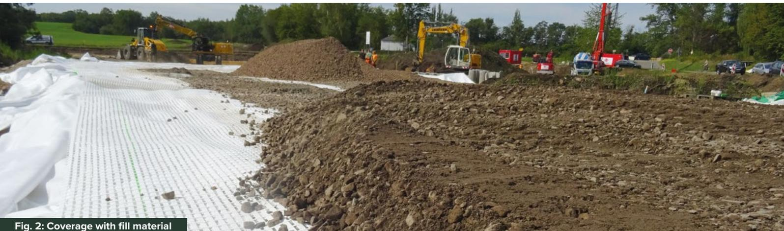
**Fig. 2: Coverage with fill material**
